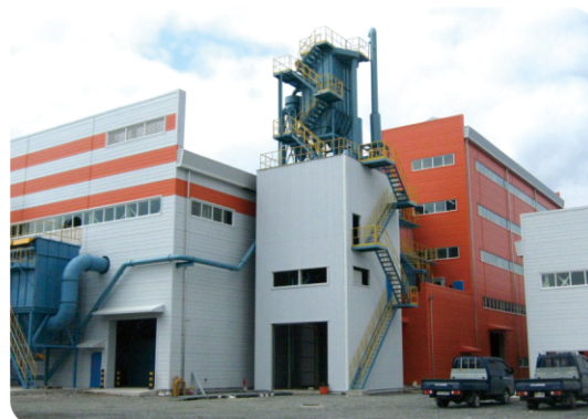
Final Dust can be loaded on the disposal truck by loading device.
