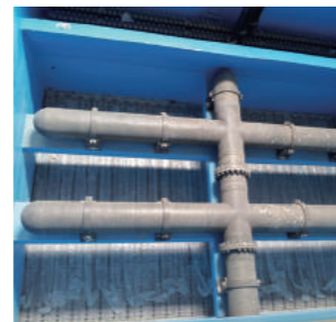
Perforated Drain Piping (for collection)
