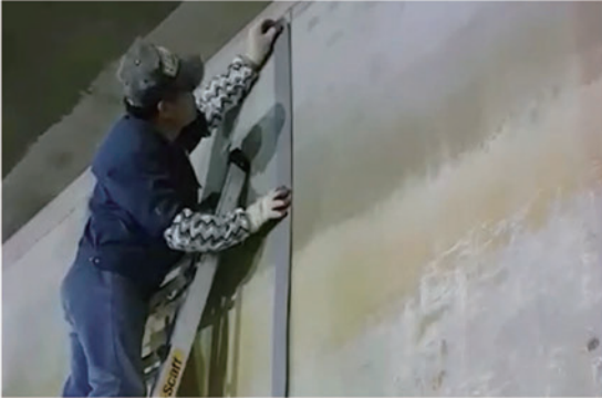
01 Attach silicon pad to the concrete wall
