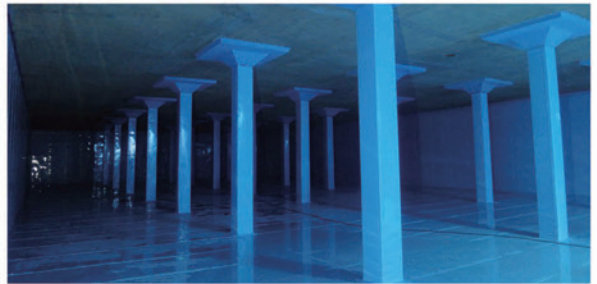
Okdong water reservoir, Andong (15,000 ton)
