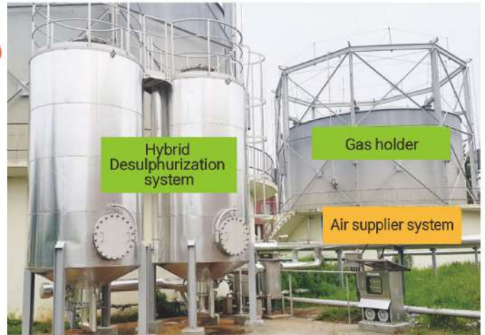
Example of Biogas Purification System
