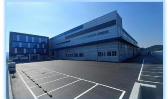
2) NEW Factory 2020 Installed (DAEGU-CITY)
